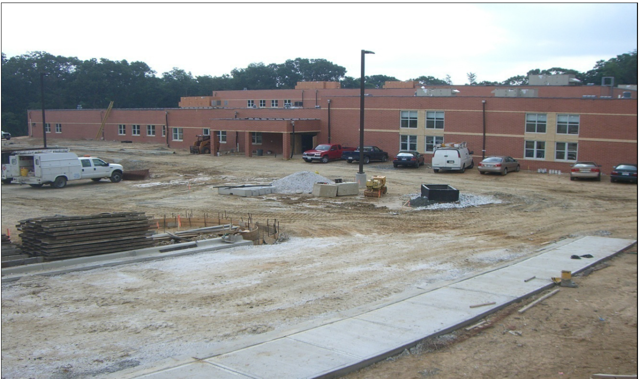
Building Exterior at Main Entrance
